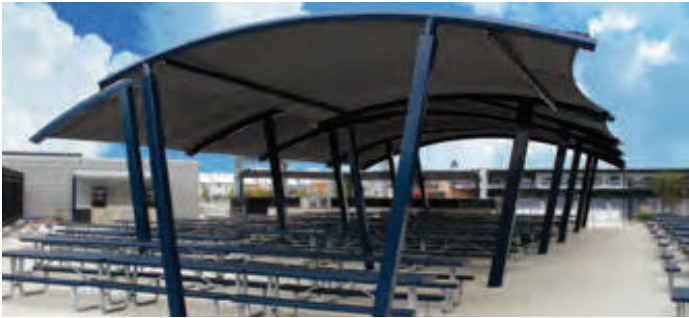
Stadium Concession Area
