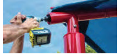
STEP 2: Use a wrench or power drill (with appropriately sized socket) to loosen the tension by rotating the drive nut. Remove fabric.
